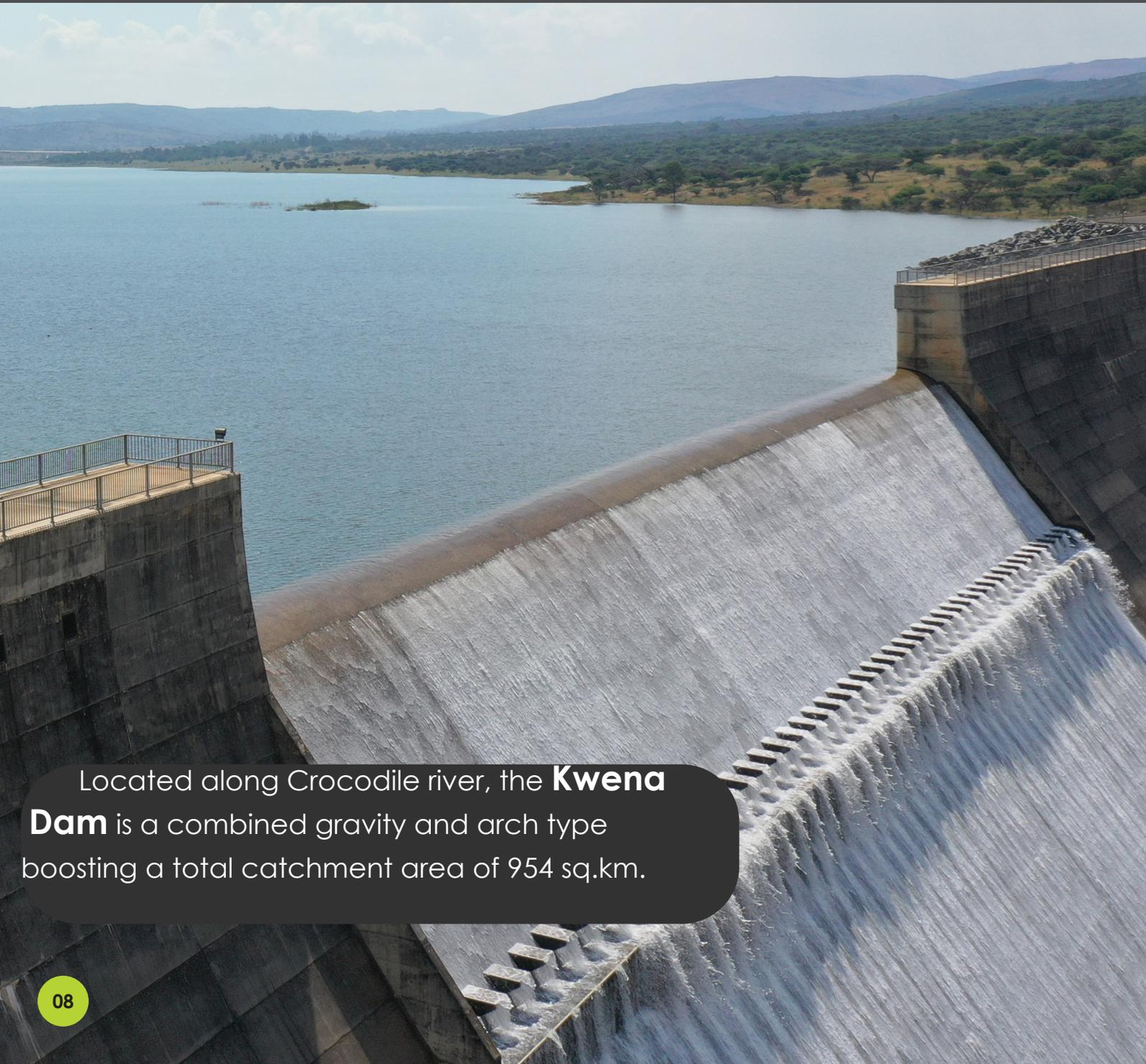
Located along Crocodile river, the **Kwena Dam** is a combined gravity and arch type boosting a total catchment area of 954 sq.km.
