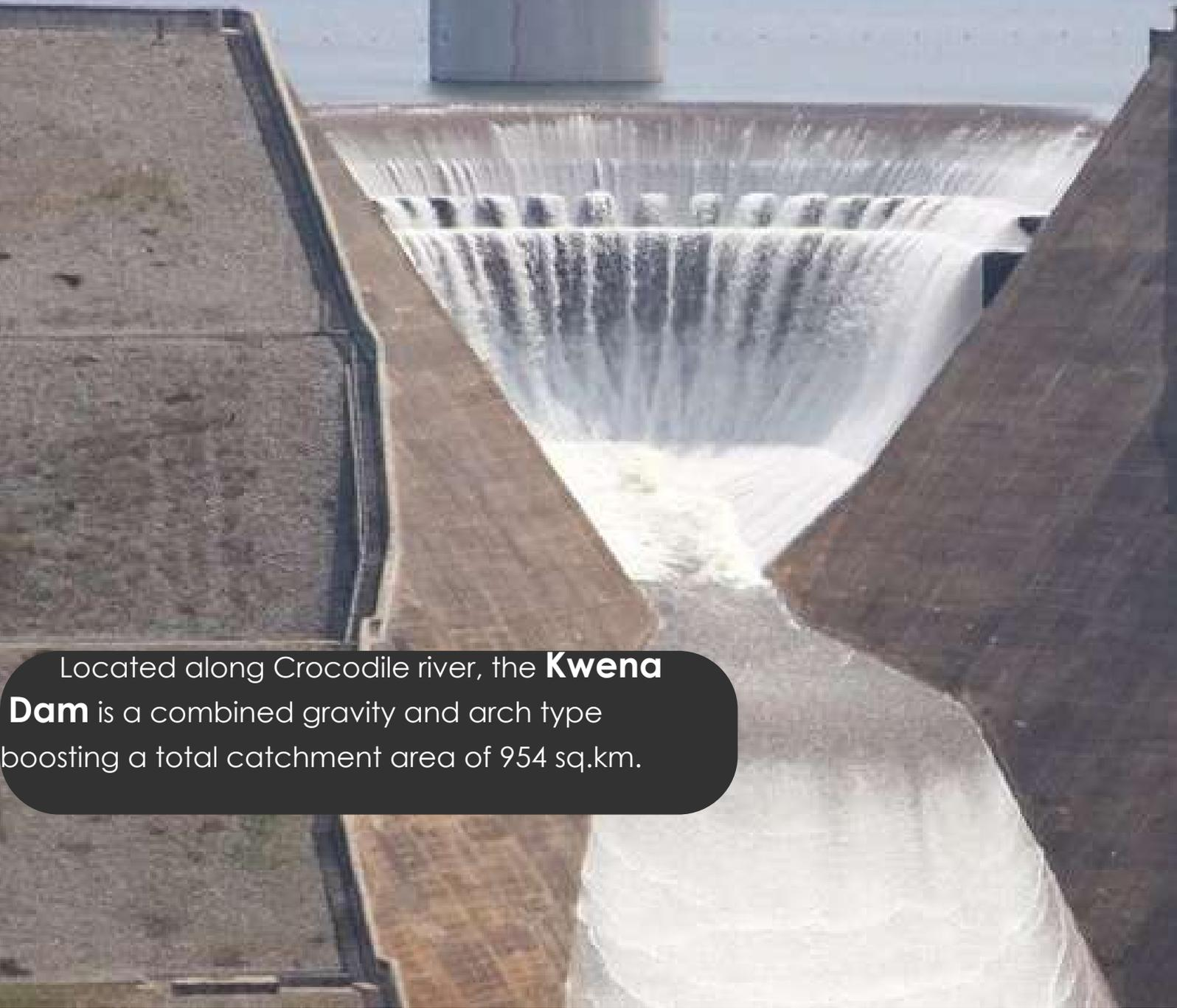
Located along Crocodile river, the **Kwena Dam** is a combined gravity and arch type boosting a total catchment area of 954 sq.km.
