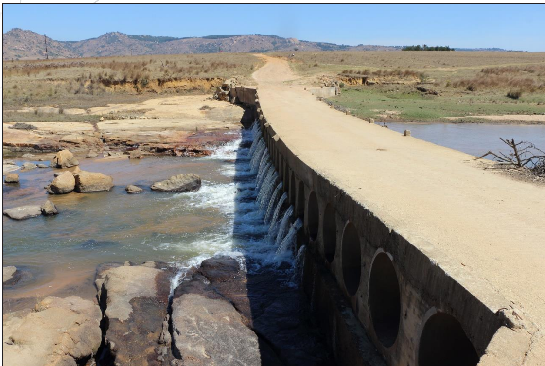
Figure 50. The bridge is an obstruction to the movement of fish during low flow conditions (9 September 2019, G Diedericks).
