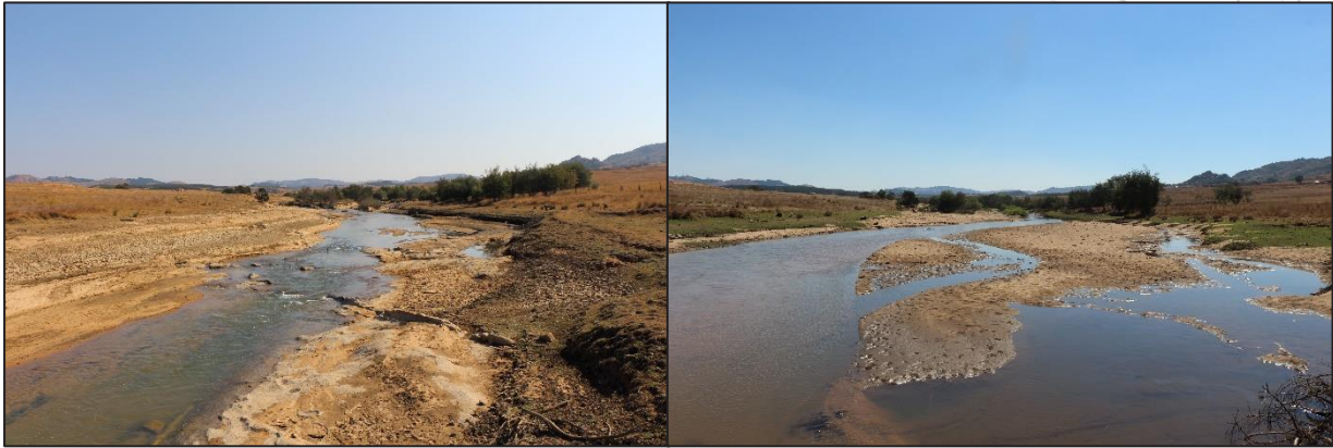
Figure 48. The photo on the left was taken upstream from the bridge at W5MPUL-VELAB on 23 July 2015, and the one on the right from the same spot 09 September 2019. A blocked culvert designed too small and is impounding the river above the crossing, with increased sediment deposition.
