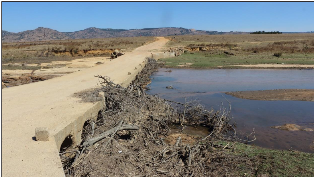
Figure 49. Small culverts at the W5MPUL-VELAB blocked with logs and debris, increased deposition of sand and organic material. The water level overtopping during high flows has effectively been raised, increasing downstream bank and bed scouring (9 September 2019, G Diedericks).
