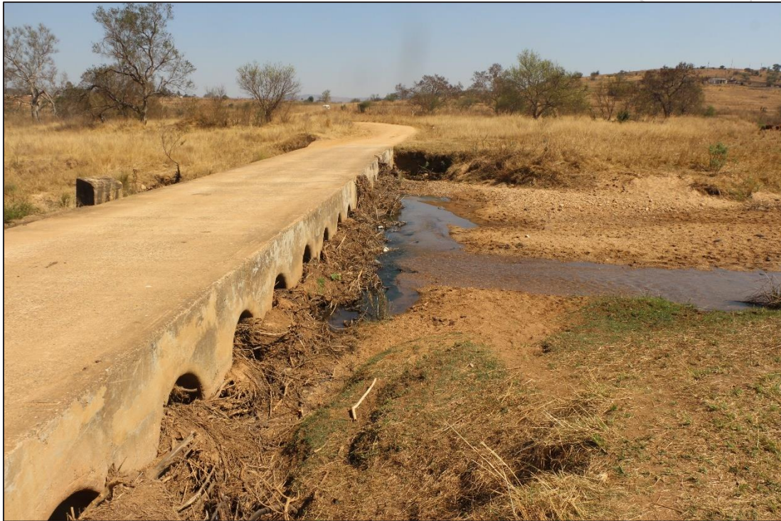
Figure 41. Culverts are blocked with organic debris, increasing deposition of sand above the crossing, and causing overtopping and downstream bank scouring during high flows (22 August 2019, G Diedericks).
