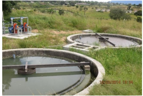
b. Humus tanks with pumps that are not working
