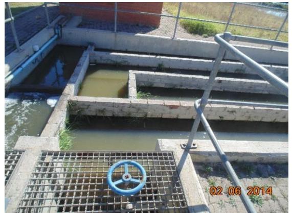
d. Chlorination channel full of floating sludge
