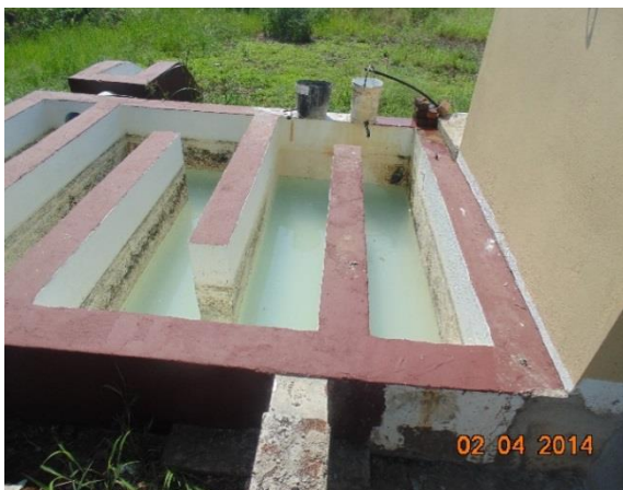
c. Chlorine channel with no outflow; only clean water
