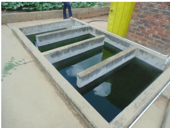
c. Chlorination channel with no disinfection taking place
