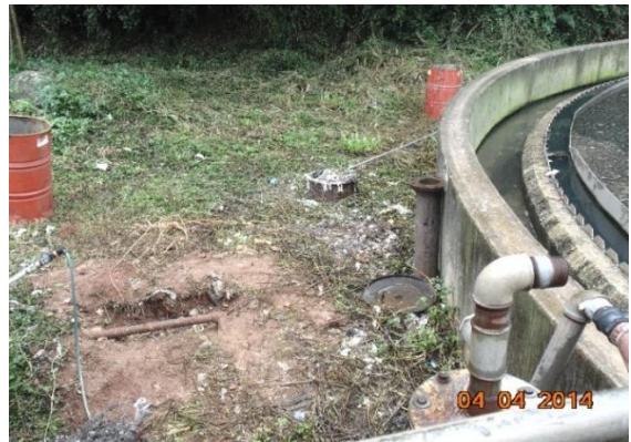
d. Improperly disposed of screenings next to the clarifier
