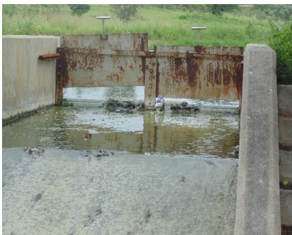
a. Scum and sludge from the final pond
