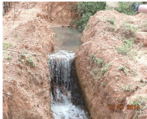
b. Broken manhole inflow into the inlet
