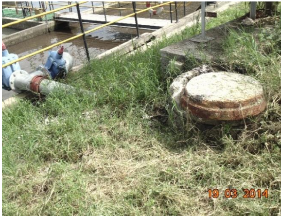
a. Traces of manhole overflow
