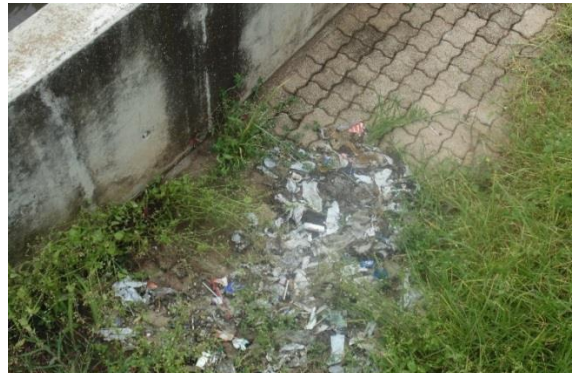
d. Screening deposited next to the aeration basin
