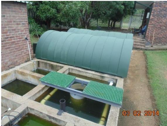
a. Plant not in operation as it does not receive or discharge sewage
