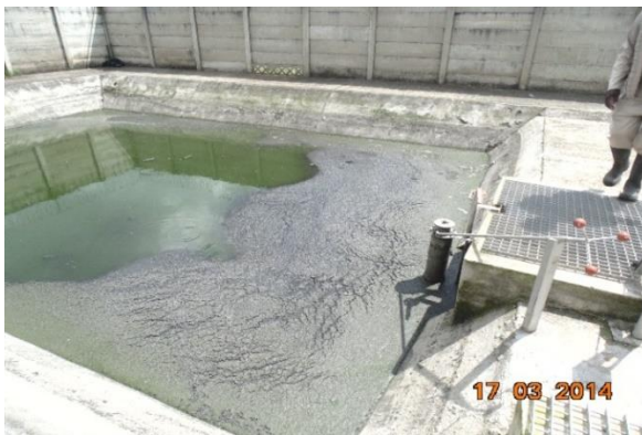
c. Drying bed and the non-functional sludge pump
