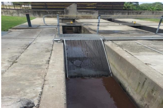
a. Inlet free of debris and equipped with automated screening remover
