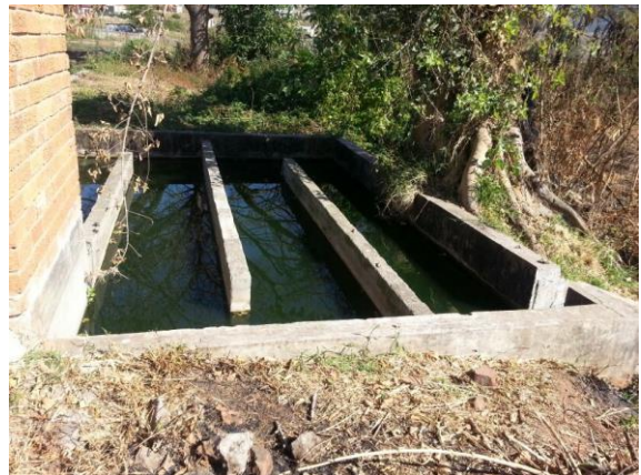
d. Chlorination channel with no disinfection
