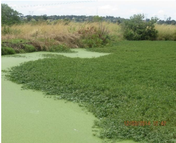
a. Primary pond overgrown with reeds
