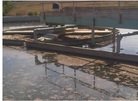
b. Clarifier full of sludge
