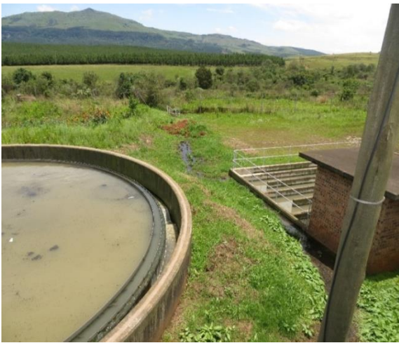
c. Overflow to the emergency pond
