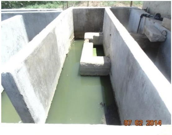
c. Chlorination channel with floating sludge
