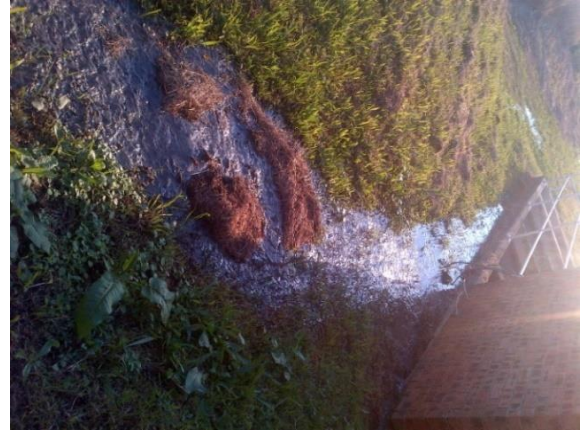
b. Overflow of raw sewage from the cracked aeration tank
