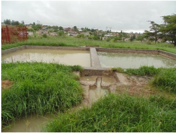
a. Inlet with collection sumps
