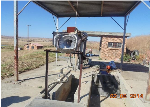
a. Mechanical screens not working
