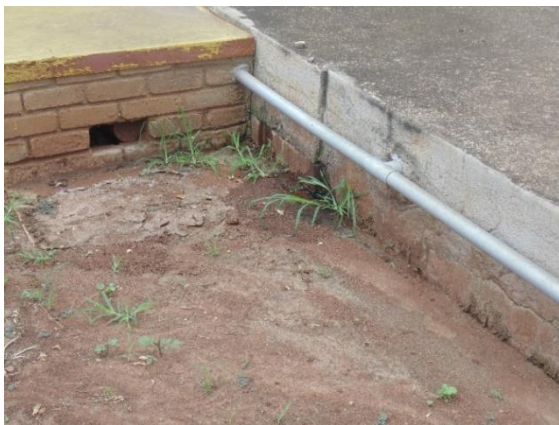
a. Traces of sewage from the bio-filters
