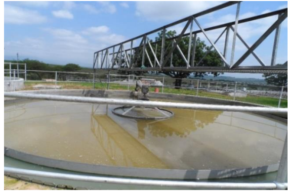
b. One of the three settling tanks
