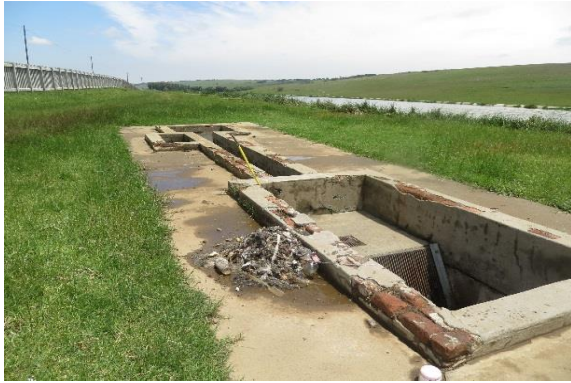
a. Screenings disposed of next to the inlet
