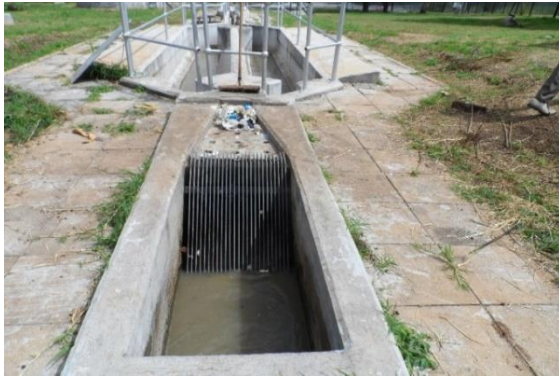
a. Screenings on the inlet
