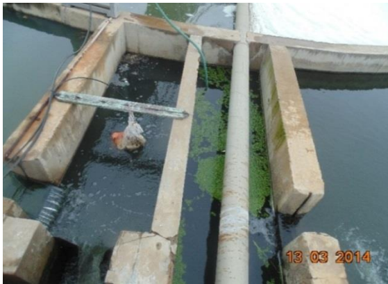
c. Some algae growing in the chlorination channel
