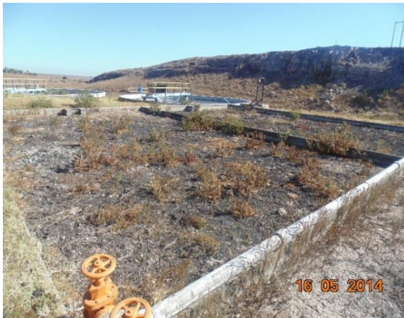
d. Drying beds no longer in use
