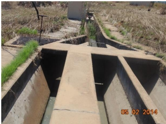
c. Grit channel overgrown with grass
