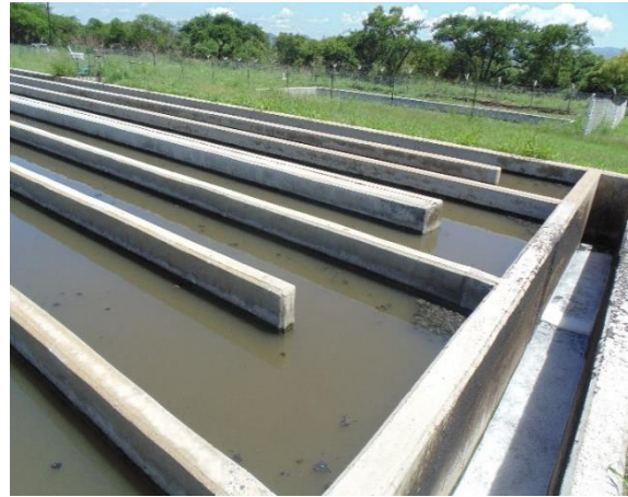
b. Chlorination channel full of floating sludge
