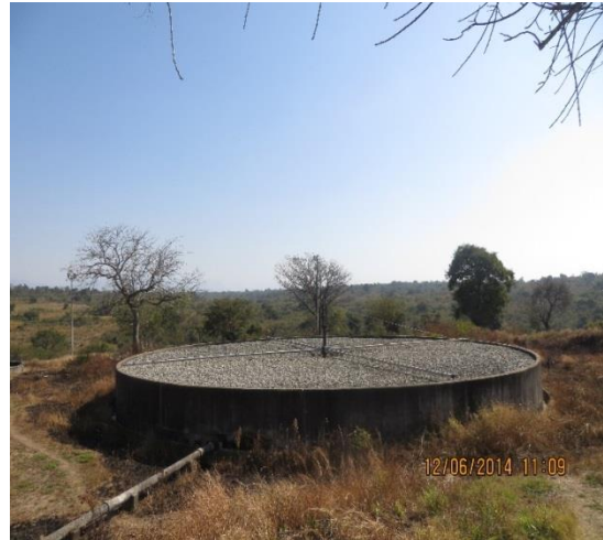
b. Non-functional bio-filter
