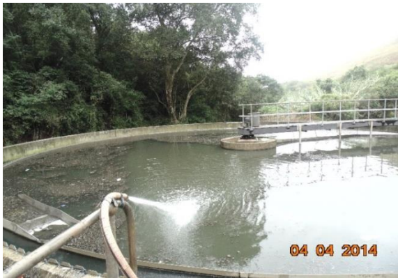
c. Pipe is installed to clean floating sludge in the clarifier
