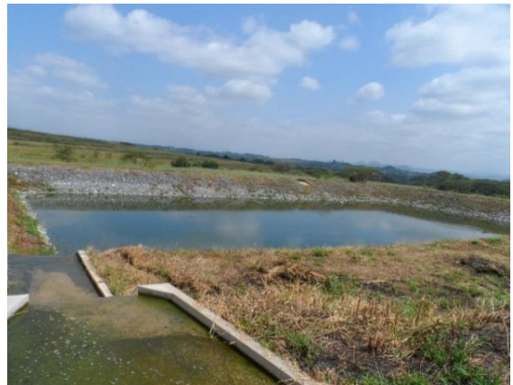
d. Final effluent disposed of in maturation pond
