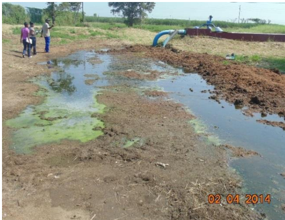
a. Sewage overflow next to the inlet pipe
