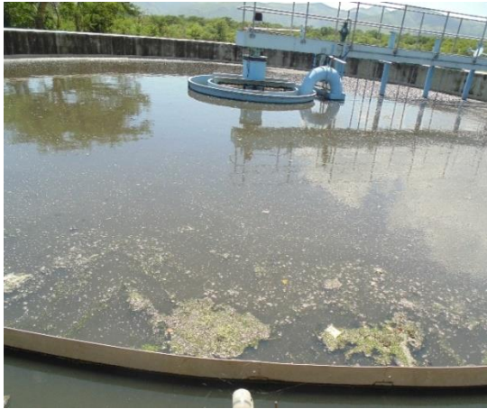
a. Clarifier full of sludge
