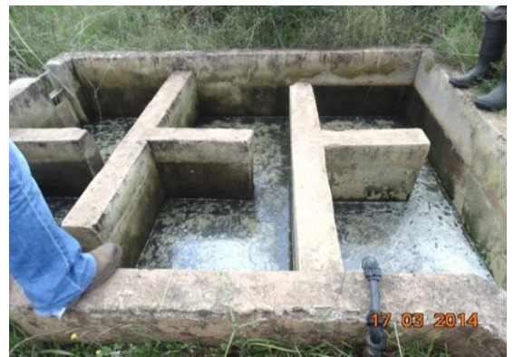
d. Chlorination channel with floating algae
