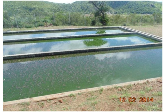
Figure 92: Pictures showing chlorination channel with floating suspended solids and drying beds full of water and sludge floating at Lebombo Border WWTW
