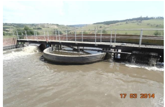
b. Aeration basin in operation with two rotation disks
