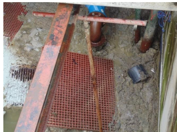
b. Pump not working and sump full of sludge
