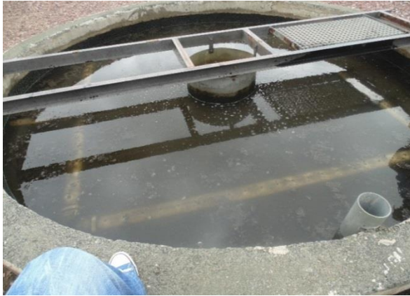
a. Humus tank with suspended solids
