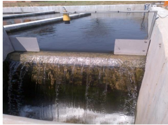
b. Effluent chlorine contact channel clear of scum
