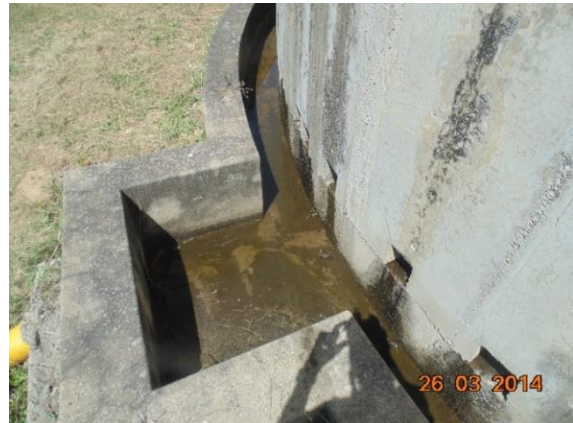
d. Overflow from the trickling filter
