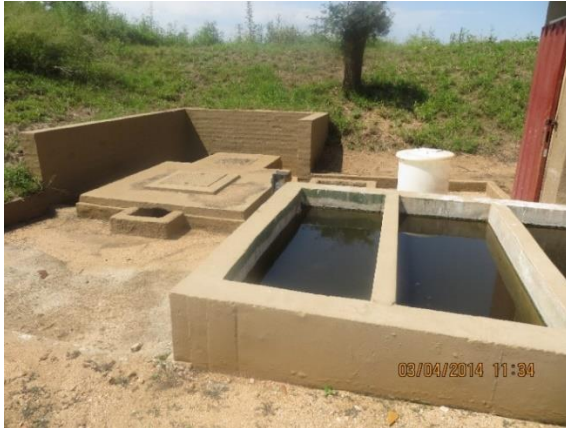
a. Chlorine dosing housing
