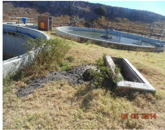
c. One clarifier in use with sludge being disposed of next to the broken clarifier
