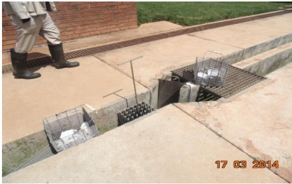
a. Inlet with proper screenings measurements
