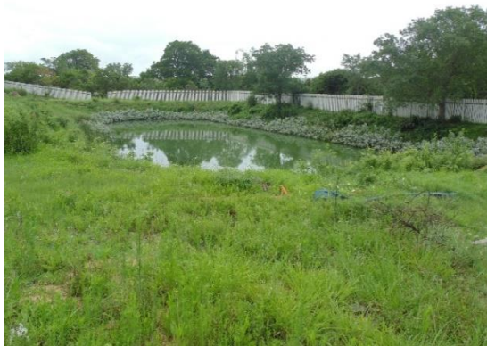
a. Emergency dam full of raw sewage
