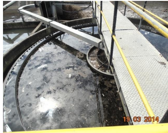
b. Clarifier full of scum and floating sludge
