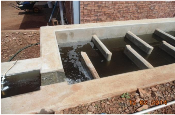
Figure 92: Pictures showing chlorination channel with floating suspended solids and drying beds full of water and sludge floating at Lebombo Border WWTW
