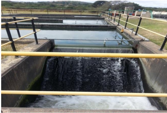
c. Final effluent disinfected and clear of scum
