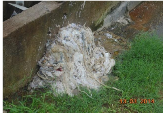
b. Screenings not properly disposed of
