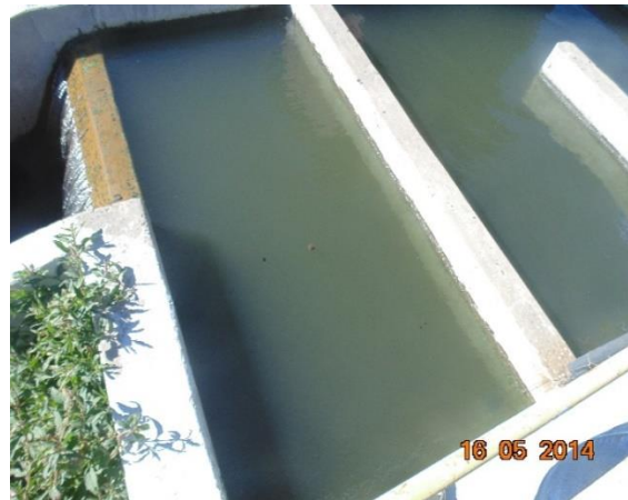
e. WWTW discharges partially treated sewage with floating sludge
