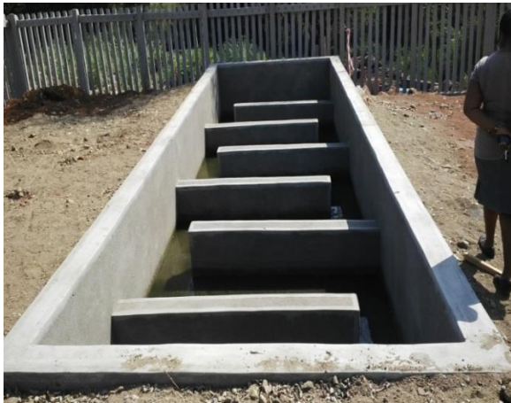
a. Disinfection chamber enlarged
