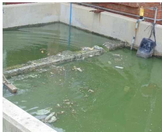
b. Chlorination channel full of floating scum and sludge
