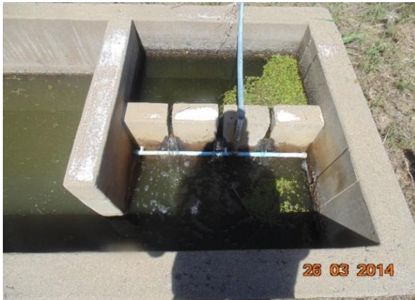
c. Chlorination channel with algae
