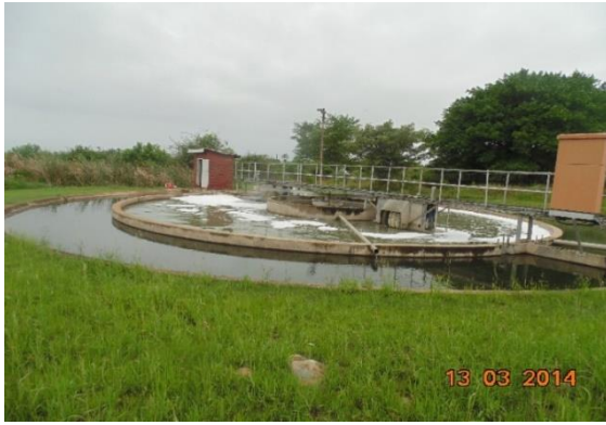
a. Aeration basin with one rotation disk working
