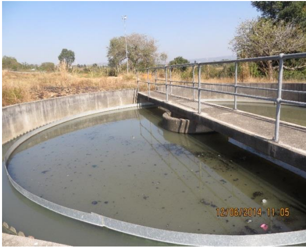
a. Humus tank with scum suspended on top
