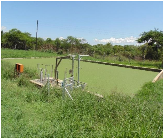
c. Drying bed full of water with algae
