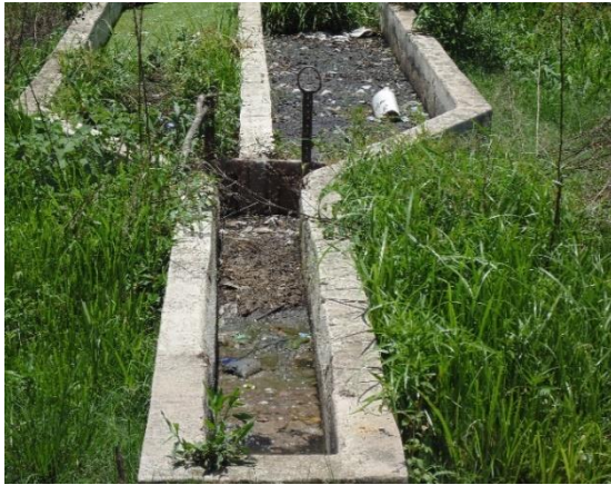
a. Inlet with scum and sludge to the septic tank
