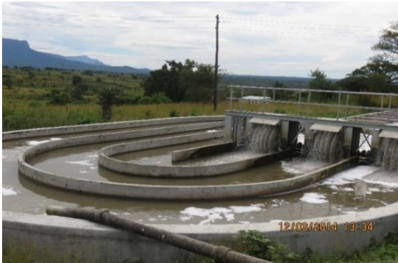
c. Treatment plant with aerators functioning well
