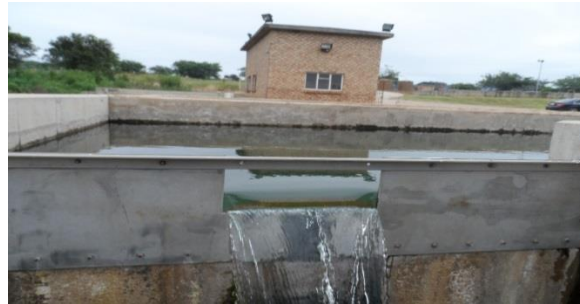
d. Final effluent disinfected and clear of scum
