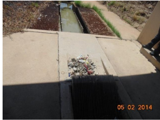
b. Screenings stored to dry up before disposal into the trenches
