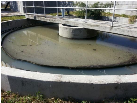
c. Humus tank full of floating sludge
