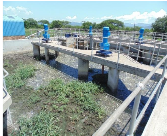
d. Aeration basin with built-up sludge
