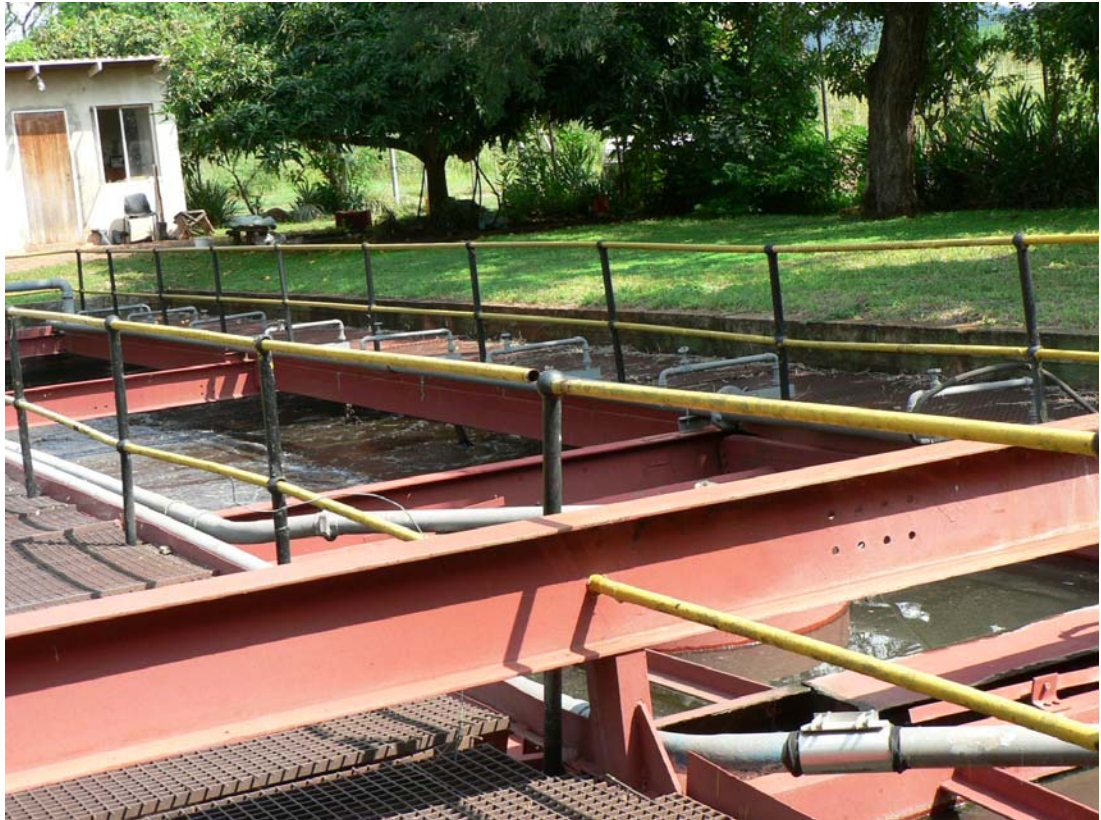
Wastewater treatment plant in EDM
