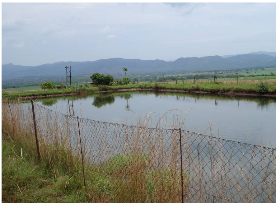
Figure 2 The first storage basin (A)
