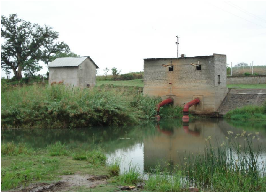
Figure 3 Nhlangu West pumphouse (left) and Ngogolo pumphouse
