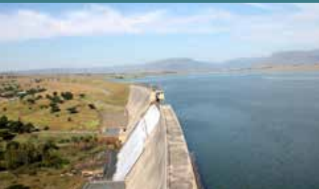
Located along Crocodile river, the Kwena Dam is a combined gravity and arch type boosting a total catchment area of 954 sq.km.
