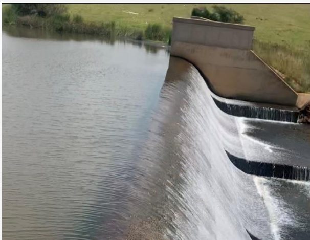
Figure 28: A photo of Boesmanspruit Dam
