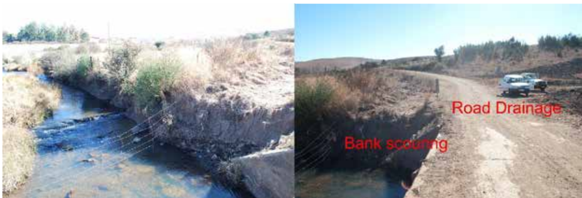
Figure 55. Stream bank scouring and high sediment inputs from the road at the stream crossing recorded at the site on the Klein Komati in 2014. The presence of invasive plant species are also evident from the photos (08 July 2014, G Diedericks).
