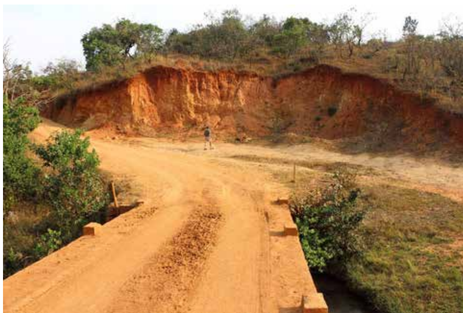
Figure 93. The road approach is steep without drainage, and a gravel source is located next to the river. This results in high sediment inputs into the river during rainfall events (20 August 2014, G Diedericks).
