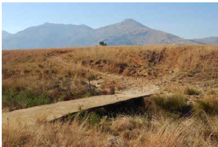
Figure 75. No road drainage at site X1TEES-WELVE, allowing loose soil to entered the river during rainfall events (11 July 2014, G Diedericks).
